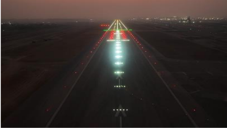
Southern Runway, Rapid Exit Taxiway, Drainage system completed, ILS26 Calibration test completed – July 2024
