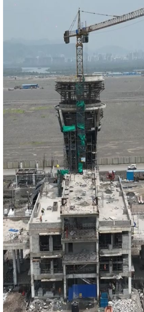
ATC handed over to AAI for instrument installation
