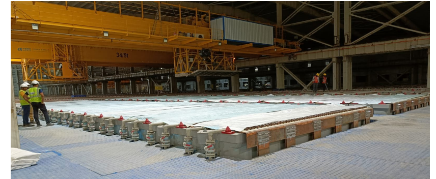
Refinery cells commissioned
